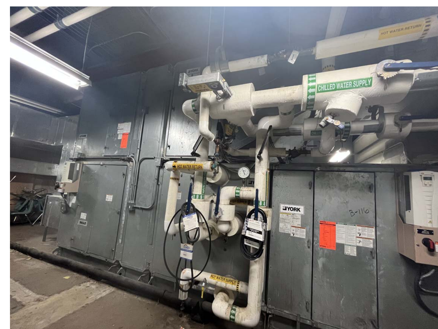
P12 PHOTO 12 - MECHANICAL MEZZANINE EXISTING CONDITIONS. MD4.2 NOT TO SCALE
