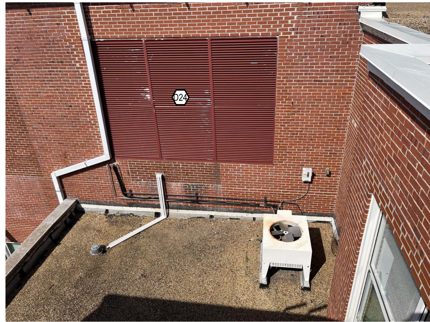
P7 PHOTO 7 - OUTDOOR AIR INTAKE LOUVER EXISTING CONDITIONS. MD4.2 NOT TO SCALE
