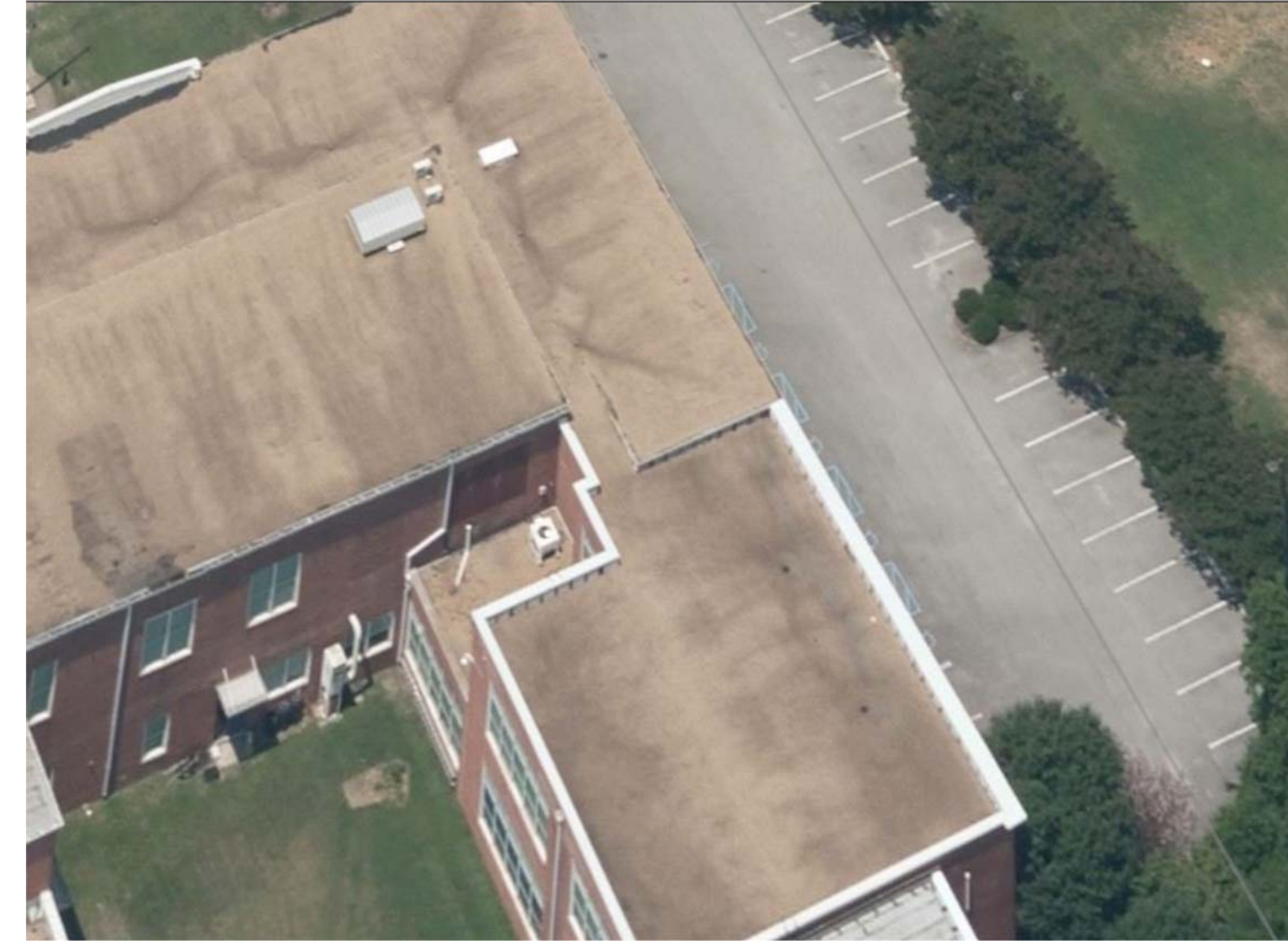
P10 PHOTO 10 - OVERHEAD VIEW OF OUTDOOR AIR INTAKE LOUVER AND POTENTIAL CRANE LOCATION. MD4.2 NOT TO SCALE
