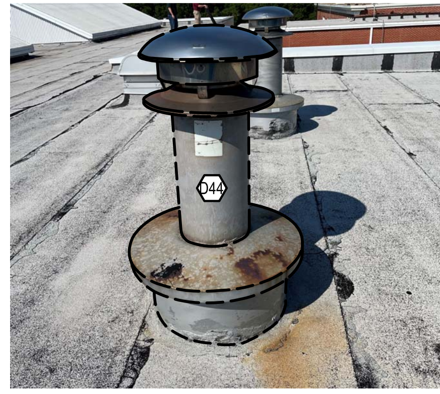
PHOTO 5 - BOILER VENT FLUE THROUGH ROOF EXISTING CONDITIONS.
